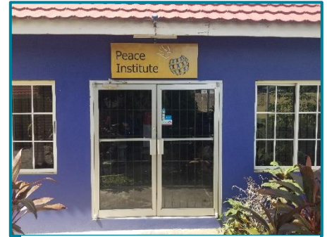
Peace Institute Sign Installed
